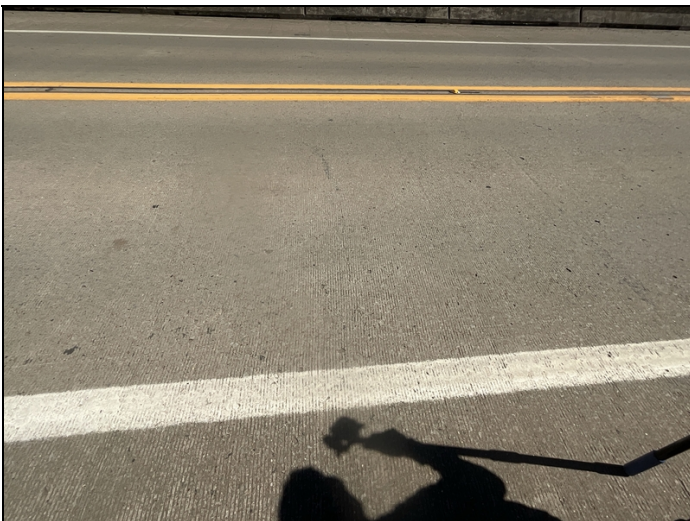
Sealable deck cracking.
