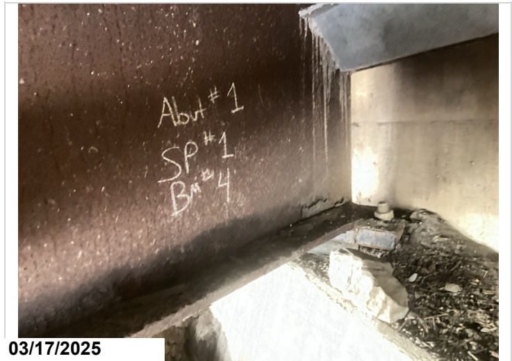
Abutment # 1, girder # 4: active corrosion with flaking rust.
