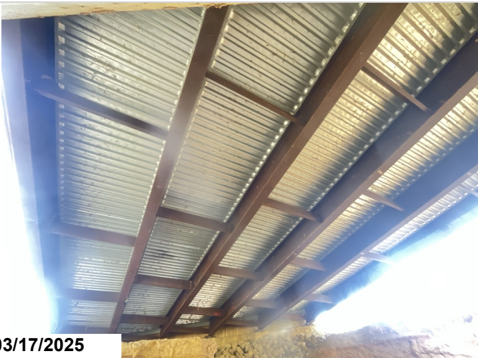
Undersurface, Span # 1: typical.
