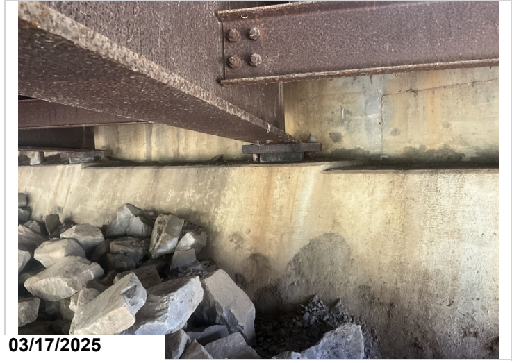
Abutment # 2, bearing # 2: active corrosion with flaking rust.
