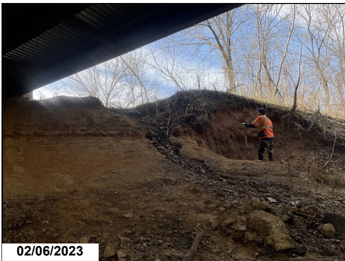
The South embankment has erosion.
