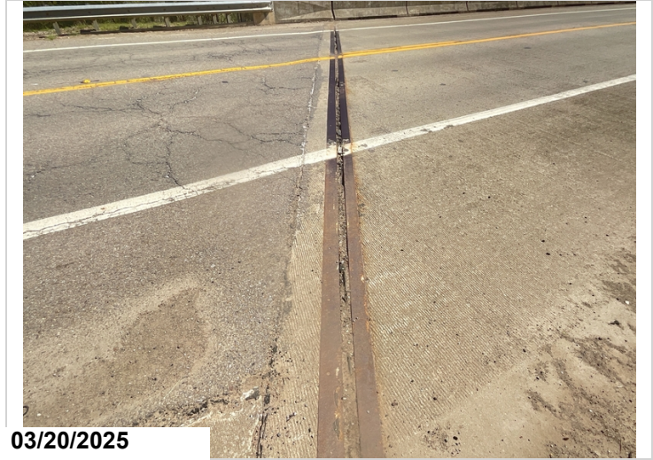
Compression Joint Seal, Abutment #2: typical.
