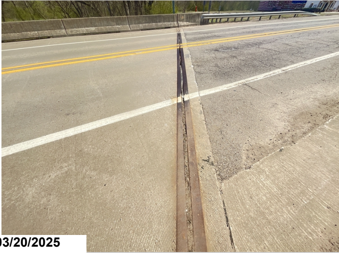
Compression Joint Seal, Abutment #1: typical.
