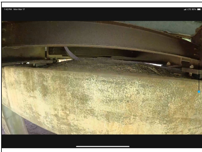
Bent # 5 debris accumulation on the bent cap.
