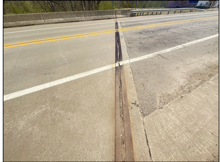
Compression Joint Seal, Abutment #1: typical.
