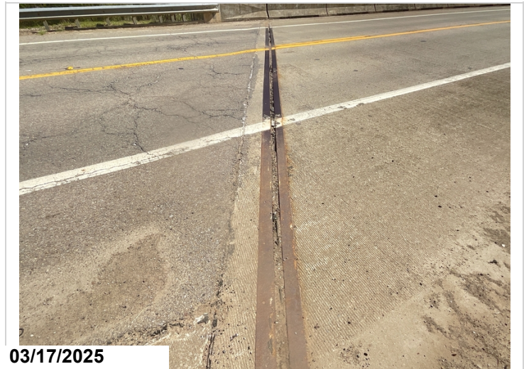
Compression Joint Seal, Abutment #2: typical.
