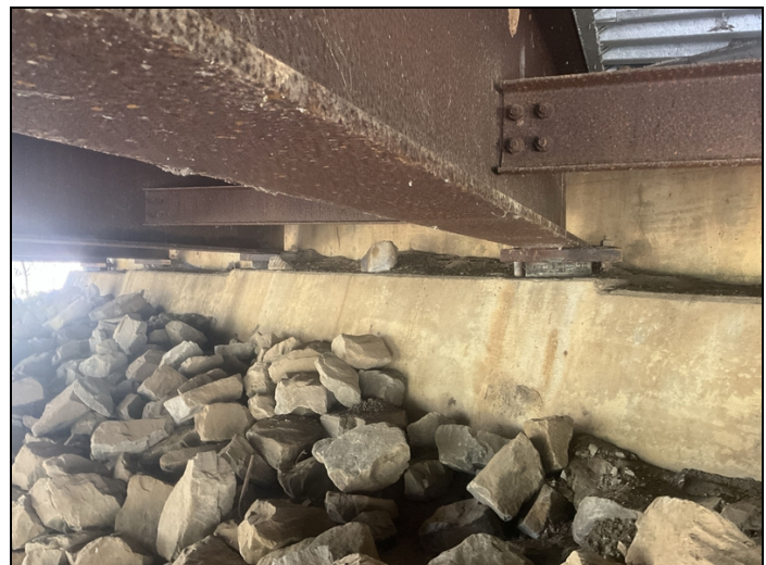
Abutment # 1 debris accumulation on the bent cap.
