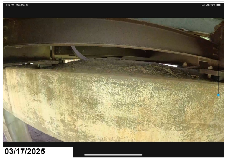
Bent # 5 debris accumulation on the bent cap.
