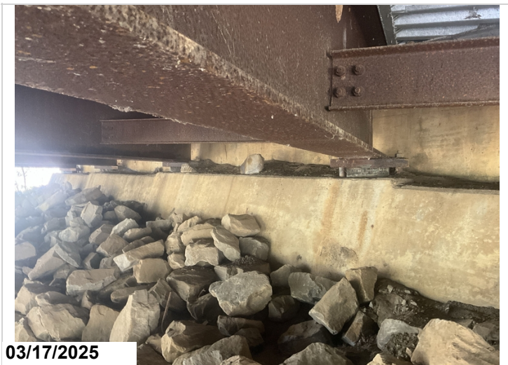
Abutment # 1 debris accumulation on the bent cap.
