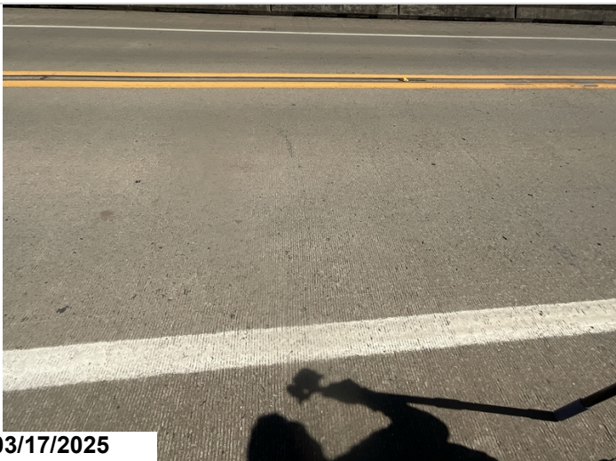
Sealable deck cracking.
