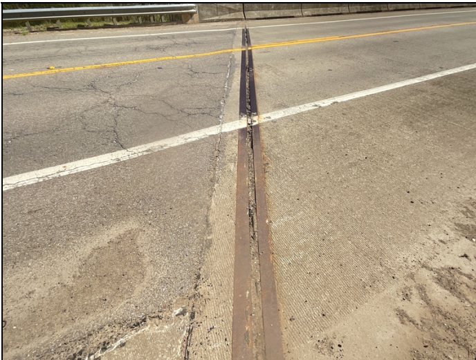
Compression Joint Seal, Abutment #2: typical.
