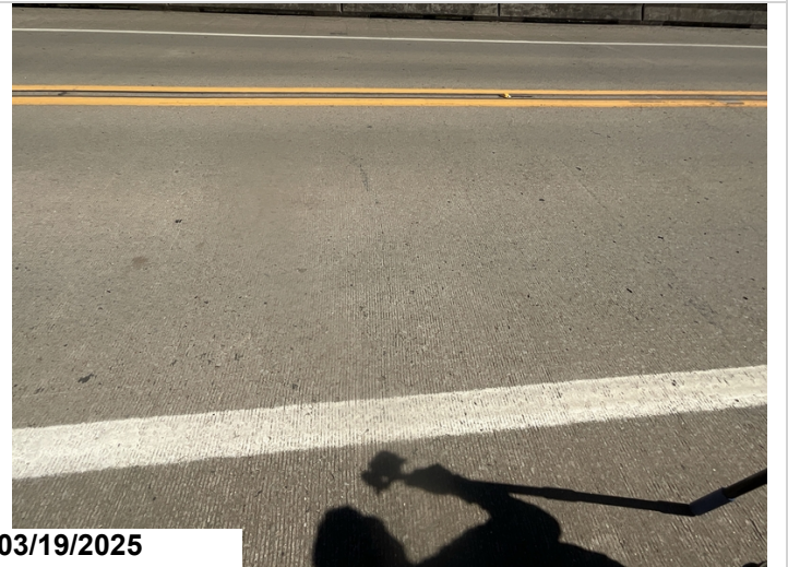
Sealable deck cracking.
