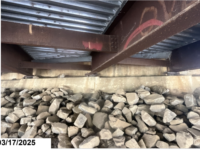
Abutment # 1: active corrosion in the bearings.
