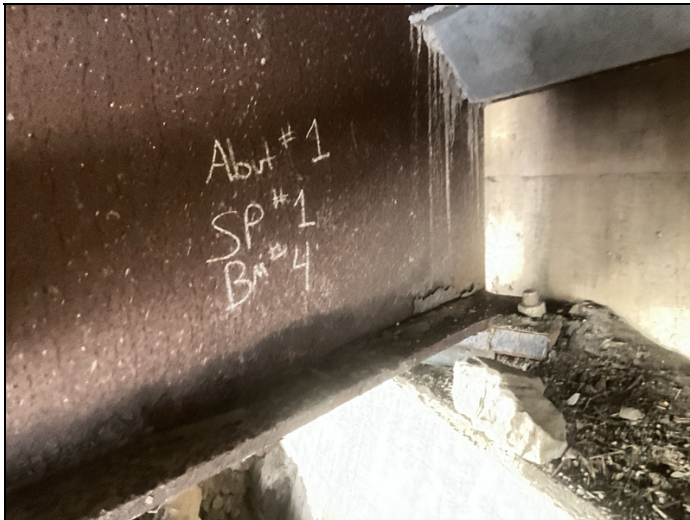
Abutment # 1, girder # 4: active corrosion with flaking rust.
