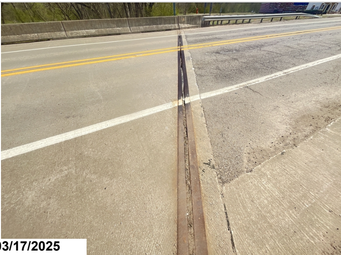
Compression Joint Seal, Abutment #1: typical.
