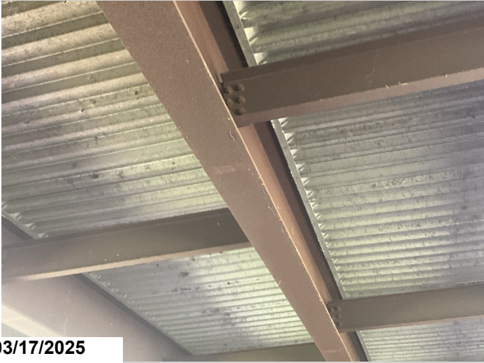
Span # 6, girder # 4: girder has a 5' areas with mill imperfections visible from the undersurface of the bottom flange at mid-span.
