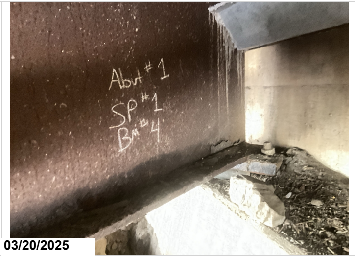
Abutment # 1, girder # 4: active corrosion with flaking rust.
